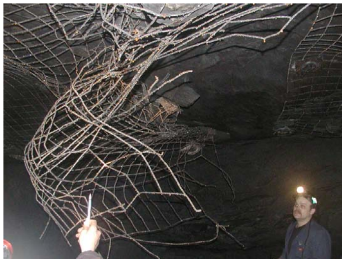
Photo 9. Wire roof mesh used as an indicator to establish apparent direction of blast forces propagating toward the top end of Old Second Left Section. Photo taken at location STA-3 on Flames and Forces Map (Appendix 5.4-1): view facing approximately N 40° E.
