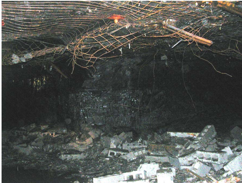
Photo 1. About 15’ outby spad 3716 (STA-2) in #2 entry. Stopping of 6” cinder block, down. Wire roof mesh partially down.
